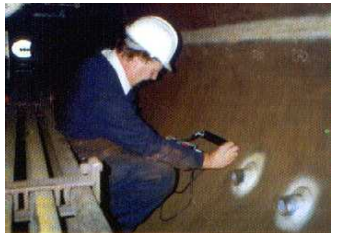
On site inspection of a steam drum
