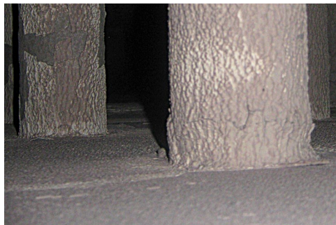
Fig 1 - Scale build-up on tube to tube plate
