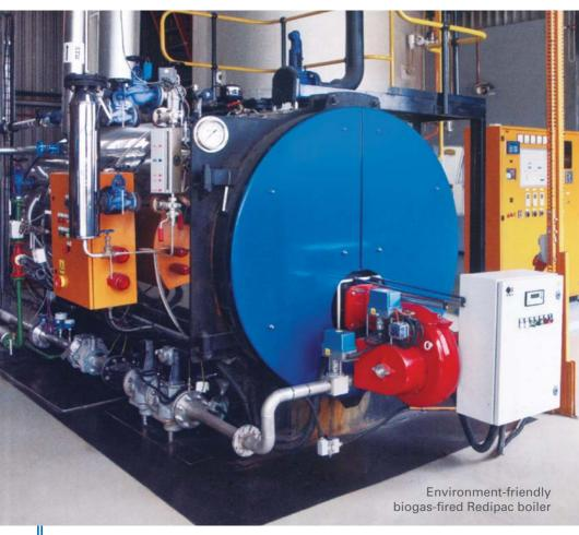
At **John Thompson** we design, manufacture, install, operate and maintain coal-, biomass-, oil-, gas- and wood-fired Package Boilers, with steam outputs from 1 to 40 t/h, for both local and international markets.
