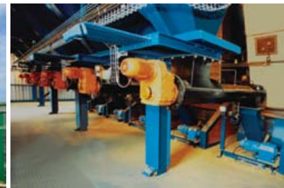
Coal & bagasse feeders
