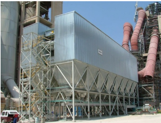
Cement kiln: Sectional units for greater cloth area
