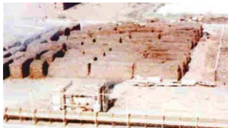
Figure 1: Fuel handling plant showing the debaler and open air storage of bales.
