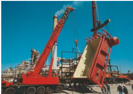
Erection of furnace front module.
